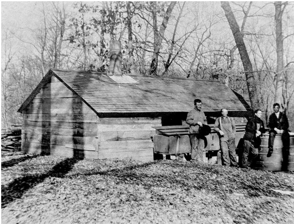
Figure 23. Open sided sugarhouse from the 1880s and 1890s built to cover a large flat pan at the Wolsfeld sugarbush. Photo courtesy of the Western Hennepin County Pioneer Association.
