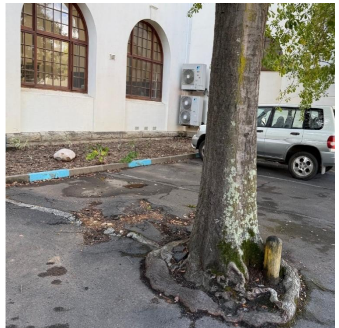
Figure 32. This water oak, growing outside the Natural Science Building at Stellenbosch University is completely surrounded by blacktop. Note how the roots are breaking up the blacktop behind the tree.
